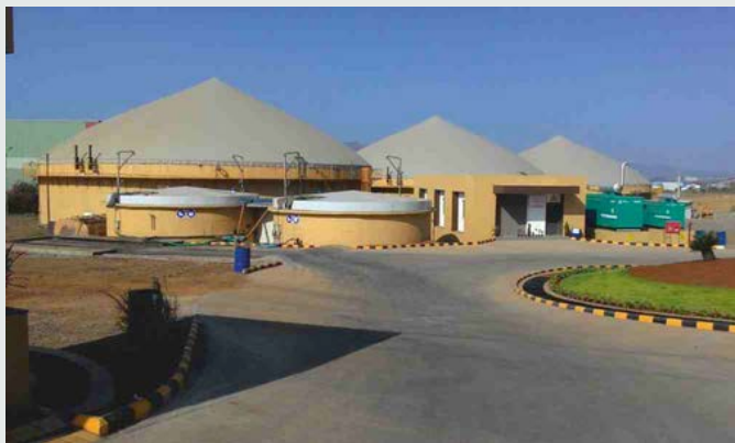
Waste Water to Biogas to Power Generation
